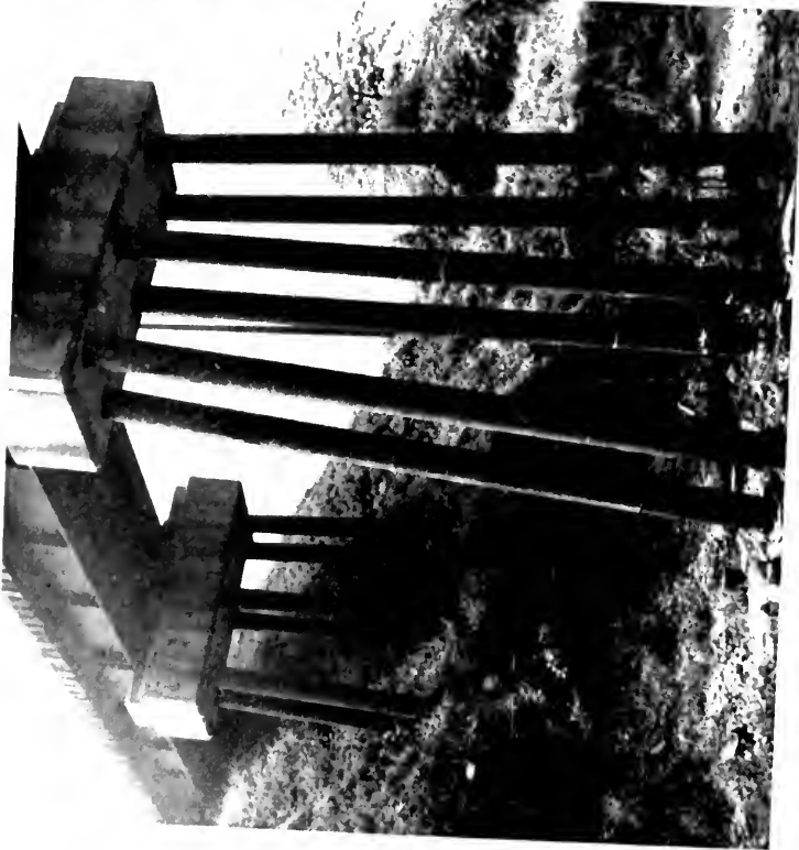
Fig. 3 (above)—View of pier 4, showing piles with timber bracing removed. Fig. 4 (right)—View of pier 3, showing new steel bracing welded to piles at 11 ft 1 in from bottom of concrete cap.
